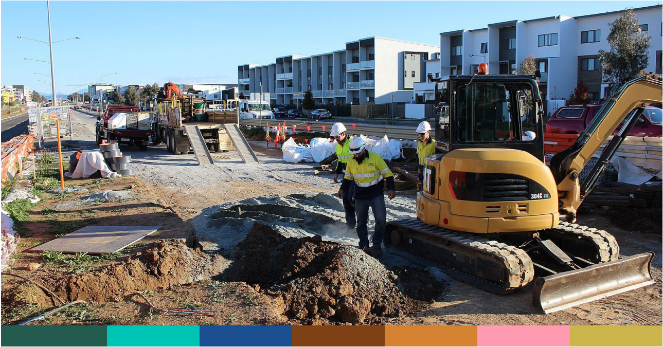
Light rail construction. Source: Wikimedia Commons
