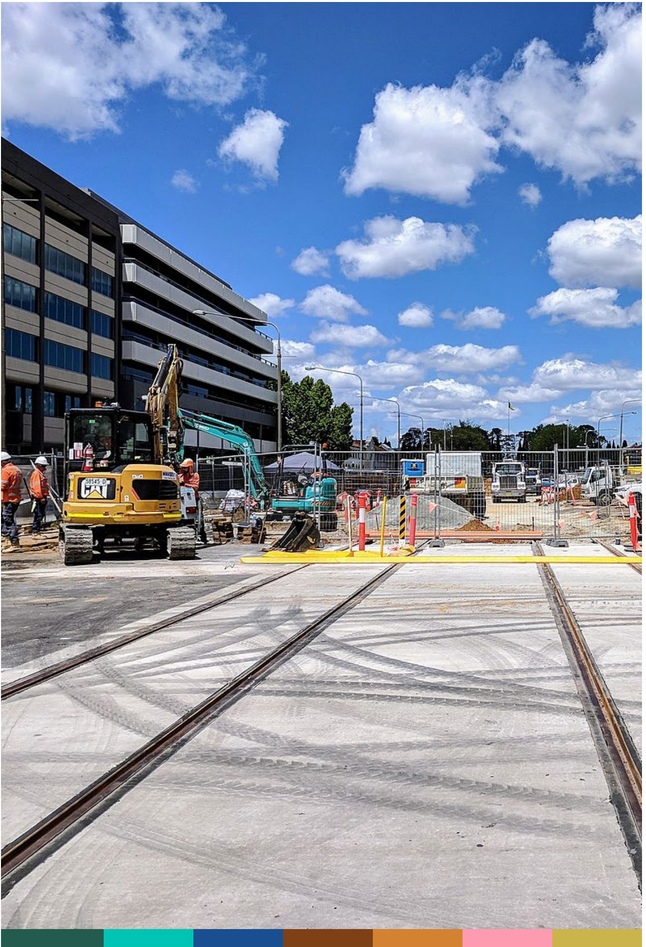
Light rail construction. Source: Wikimedia Commons
