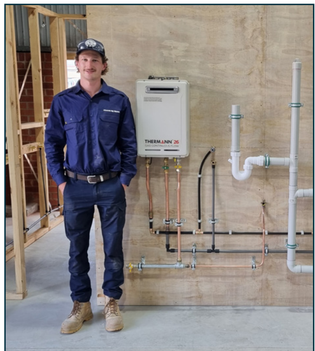
Elliot Nunn — Plumbing, WorldSkills Challenge
