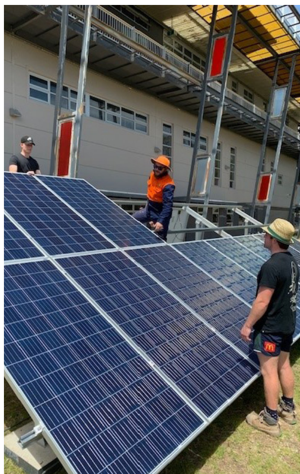
CIT students installing panels
