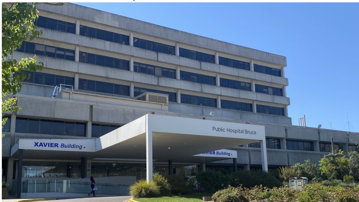
Figure 5: North Canberra Hospital
