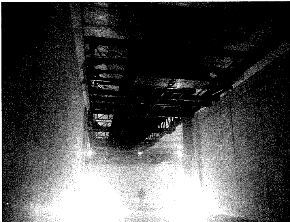
Figure 8: Example of a composting tunnel, internal view. Image supplied by technology composting provider Christiaens
