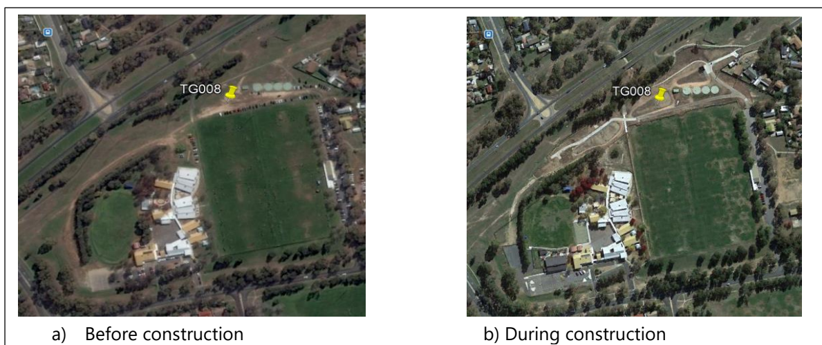
Figure 19. TG008 aerial images before and during construction
