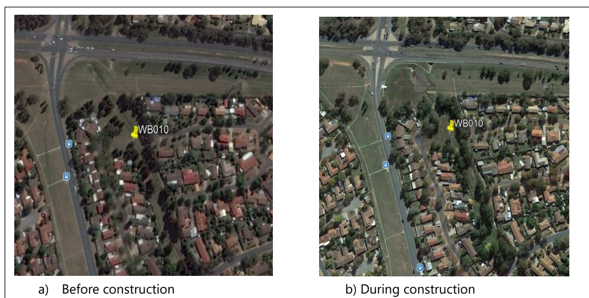
Figure 30. WB010 aerial images before and during construction
