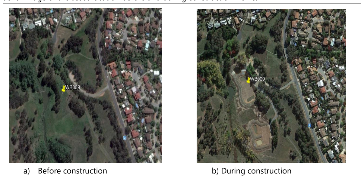
Figure 29. WB009 aerial images before and during construction
