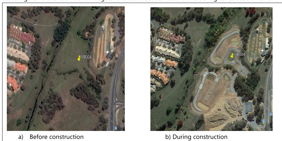
Figure 28. WB004 aerial images before and during construction
