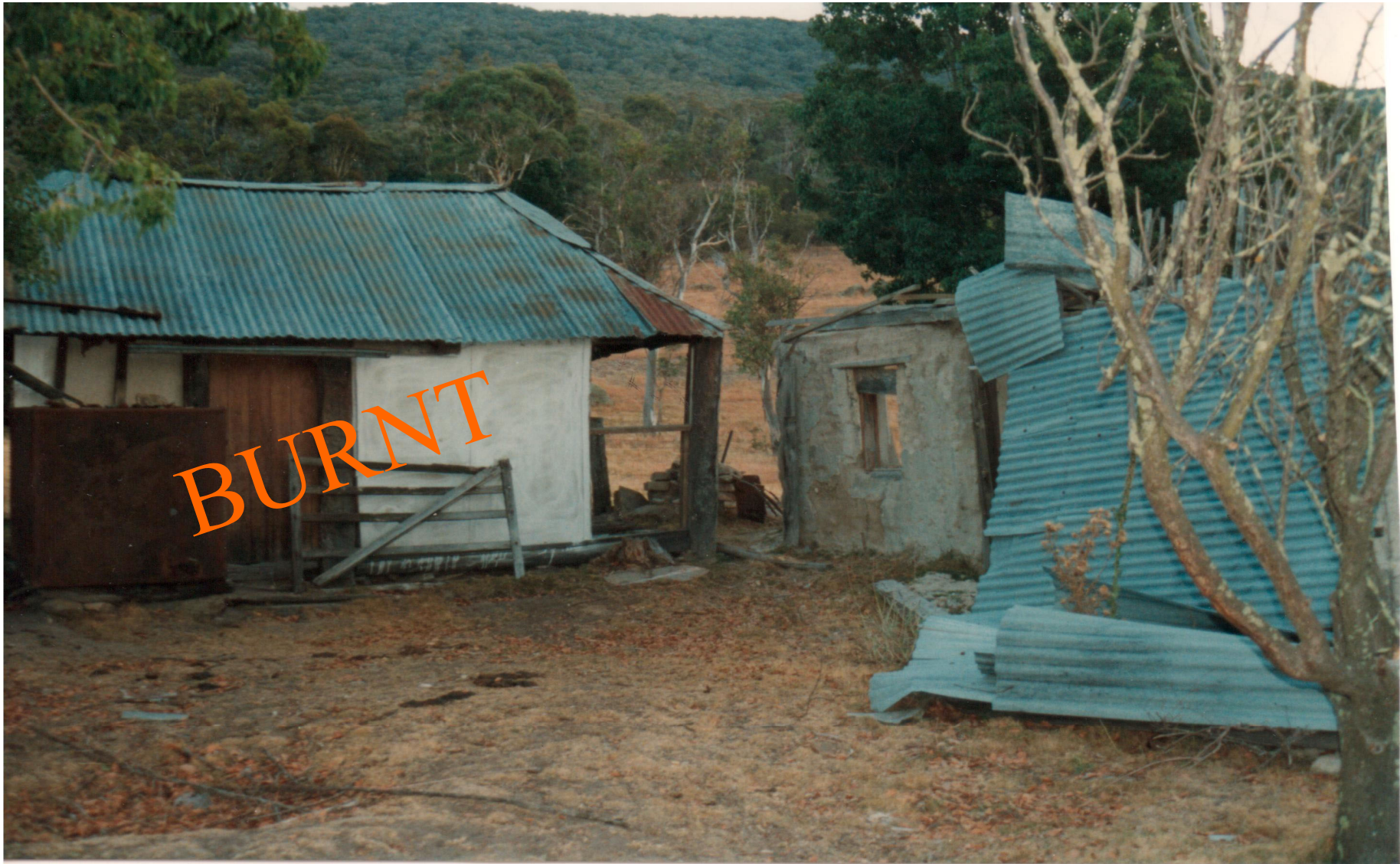
Mt. Tennent Homestead (1892 - 2003) - destroyed by bush fire
