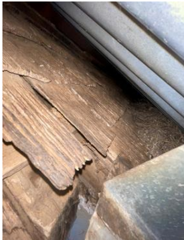
'Majura House' cottage: (above) timber shingles under roofing iron (2023 Fred McGrath-Weber); (right) interior (ERM 2013)
