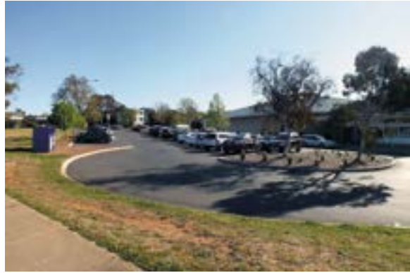
INEFFICIENT PARKING LAYOUT AND DESIGN
