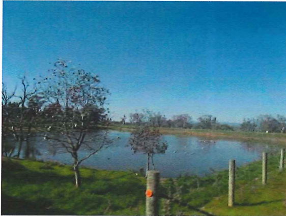
Main Dam (Block 1599)
