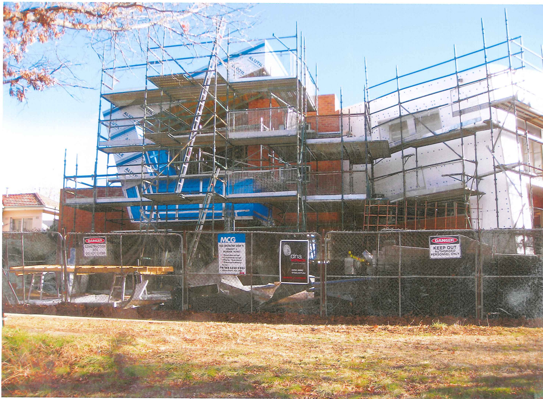
Figure 1, 32 Stuart Street, Griffith RZ1, 4 July 2012
