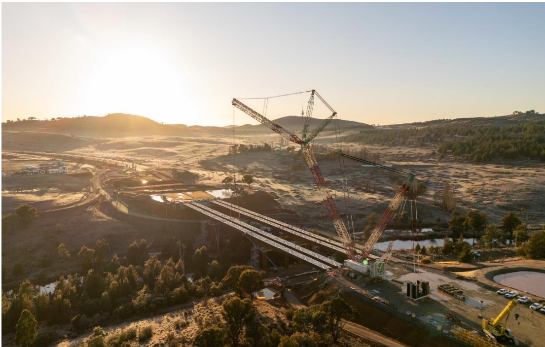
Molonglo River Bridge Lift
