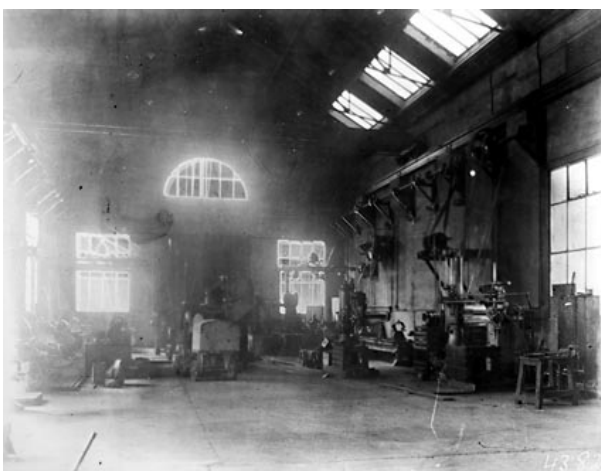
Image: Original interior of the Fitters workshop. Note the skylights in the roof that are no longer visible in the current building.
