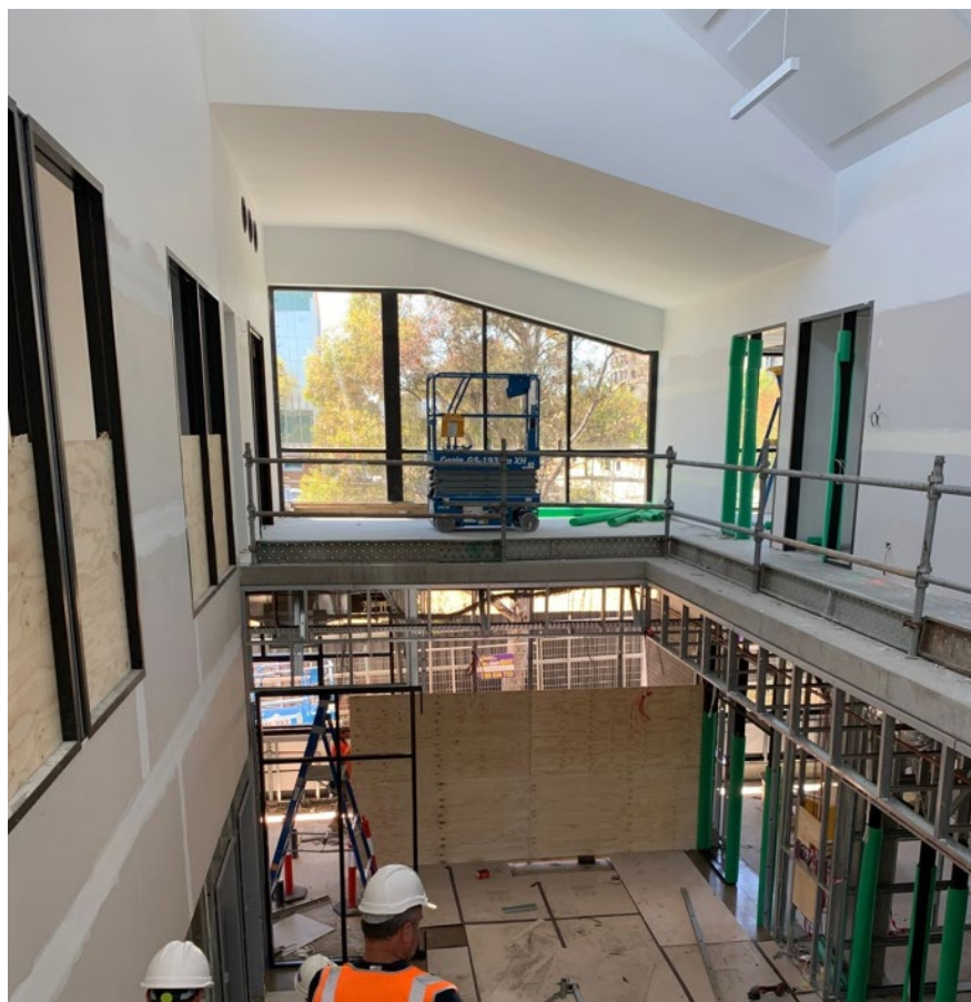
Gungahlin Community Centre - Atrium
