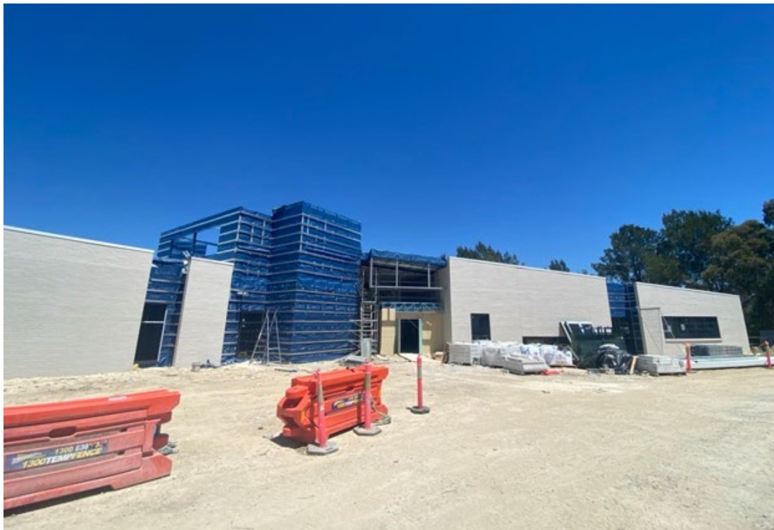
Conder Health Centre Construction
