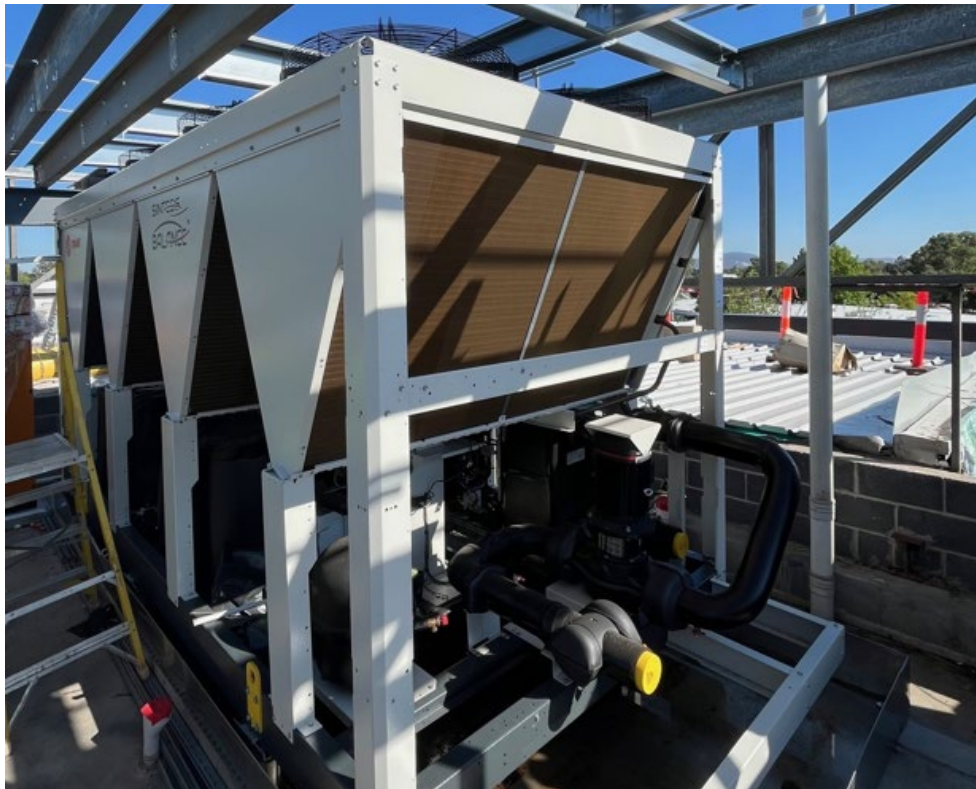
New plant at 255 Canberra Avenue
