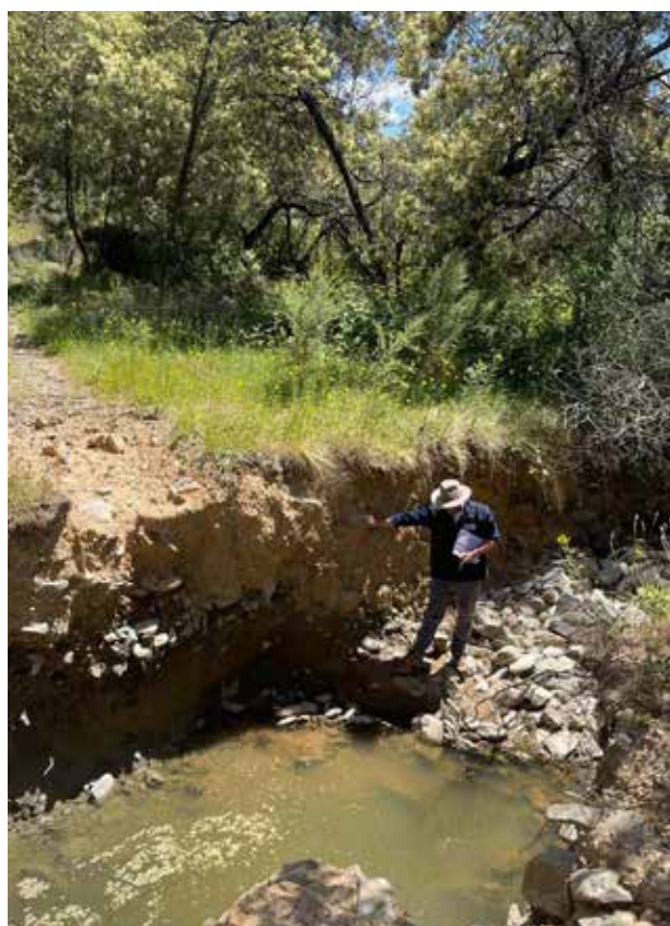
Extreme gully erosion on Googong Creek at GGG050 has cut the access trail
