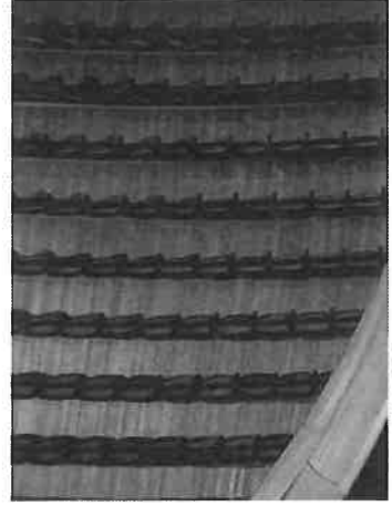
Timber Floors in stalls and balconies
