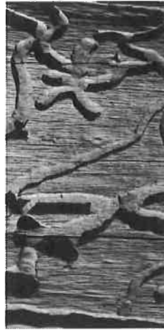
Surface texture for sound scattering
