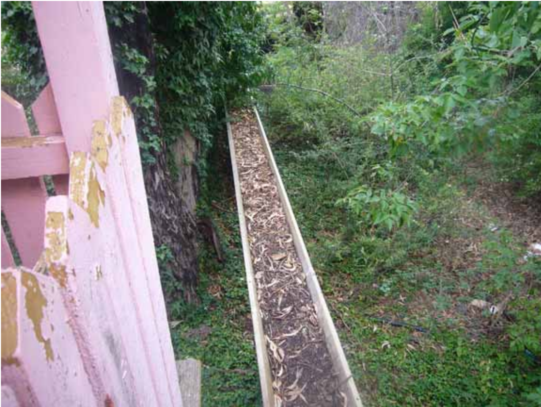
Figure 23. Mill race at the Mill House (note the neglect of the race and building).
