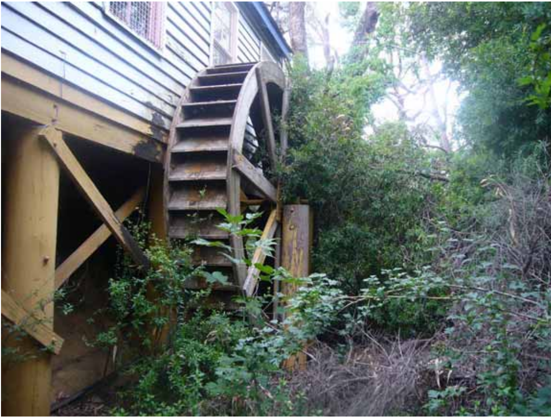
Figure 22. Mill wheel at the Mill House (note the neglect of the wheel and building).
