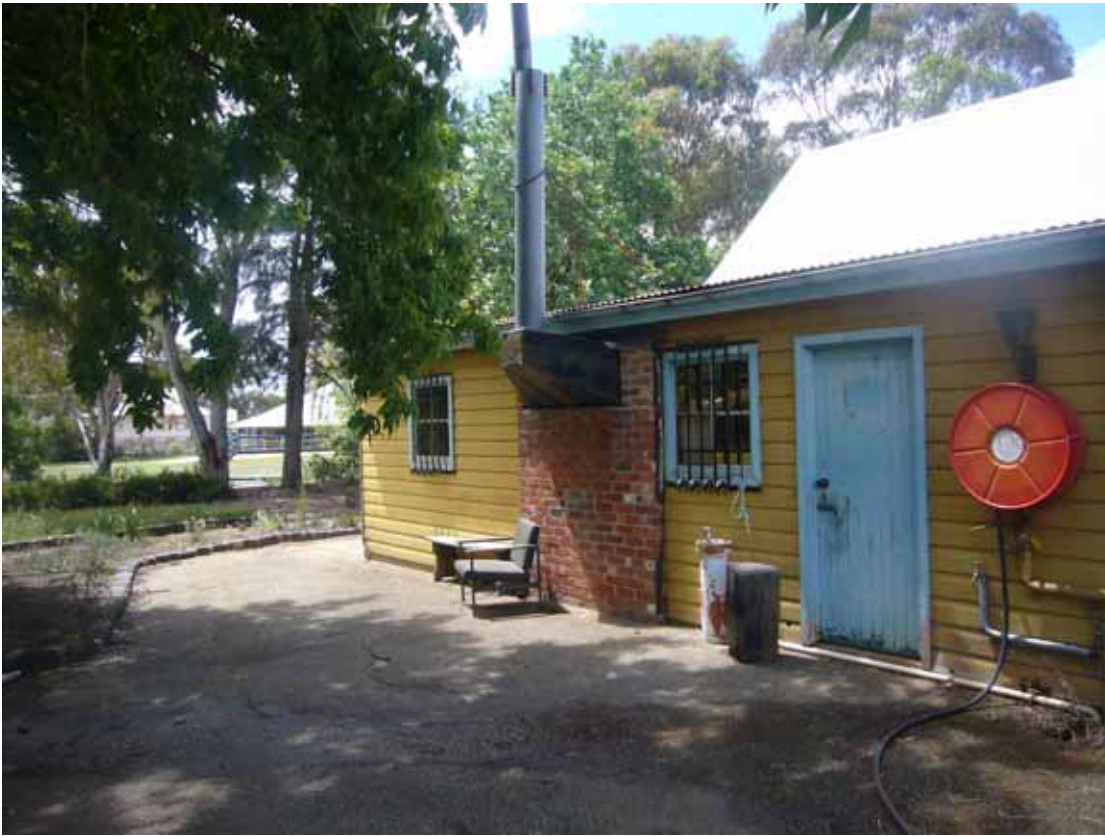
Figure 18. Side view of cottage industries shops showing the brickwork and chimney for the forge.
