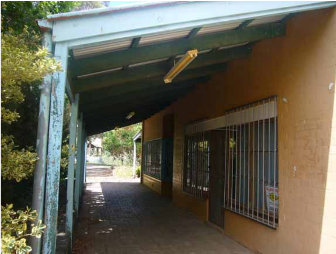
Figure 14. Front view of cottage industries building with awning. The visually inconsistent steel security grills are not original but were installed during current ownership.
