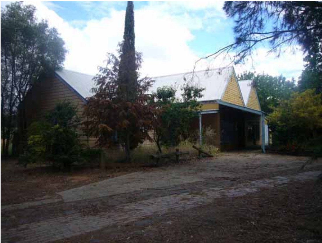
Figure 13. Cottage industries building viewed from the northeast.
