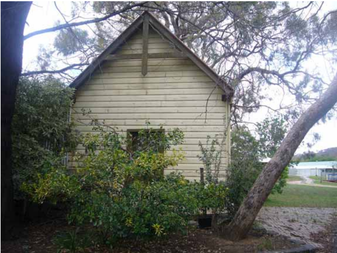
Figure 31. Possum Gully Railway Station (side view).
