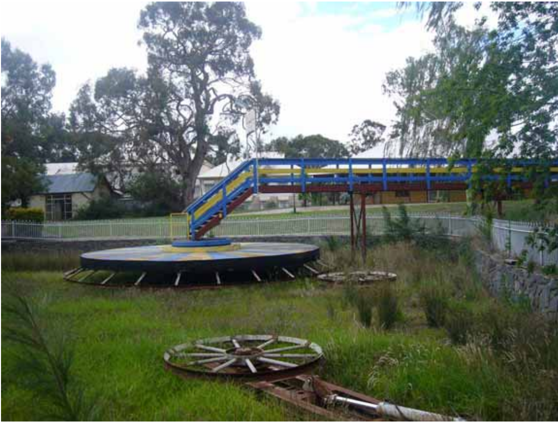
Figure 24. Boardwalk for swan ride (originally pedal boats). The inappropriate and garish colour scheme dates to the time of the failed amusement park venture (during the period of current ownership). Eight small wheels turned the steel plate platform.
