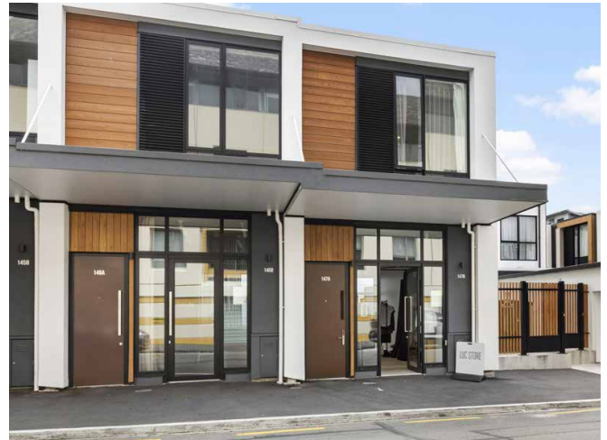
Photo 34: Generous ground floor ceiling heights allow for flexible uses such as micro-retail or a cafe.
