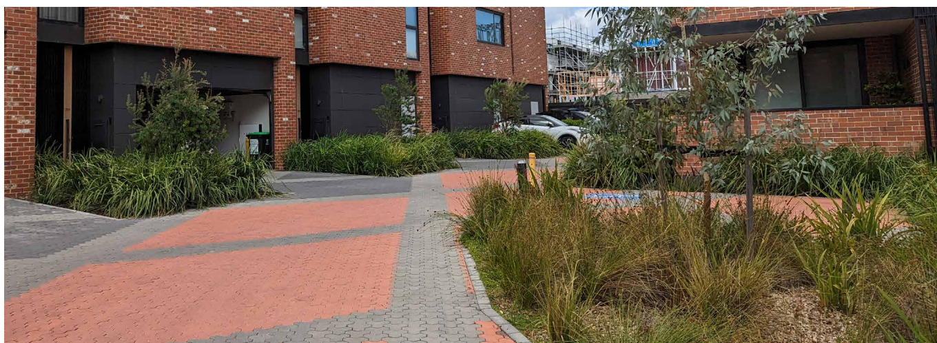
Photo 29: Permeable paving combined with green infrastructure, such as rain gardens, can help to manage runoff (reducing pollution) and reduce the risks associated with flooding and rainfall surge events.
