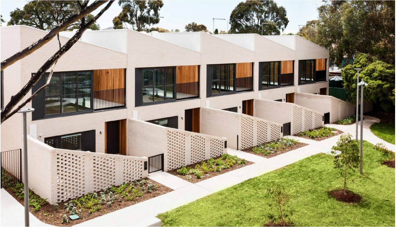
Photo 68: A building to open space creating a highly legible transition where the street is surveilled while residential privacy is maintained. Image: Social and affordable housing, Tarakan Street, VIC. NH Architects.
