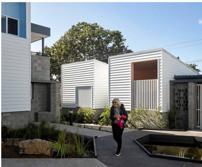
Photo 9: Integrated landscaping can enhance communal and circulation spaces for townhouse developments.
