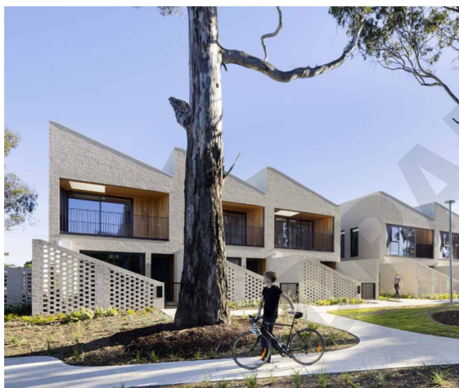
Photo 17: Balconies activate the streetscape and a consistent architectural language creates a integrated built form.
