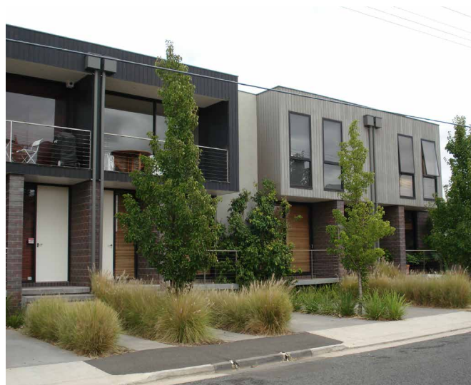
Photo 16: Architectural articulation and varied materiality can help to avoid a repetitive frontage.
