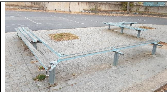
Upgrades needed to outdoor seating – due to recent vandalism
