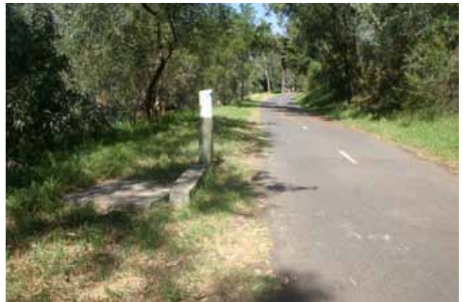
Figure 14 – It is critical that all invisible obstacles and hazards are identified or removed.
