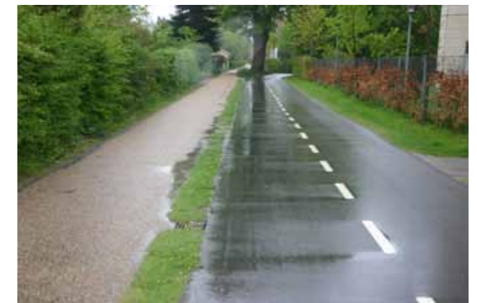
Figure 13 – Surface texture and colour are used on these paths to separate pedestrians from cyclists and to make it clearer as to which paths cyclists and pedestrians are required to use. In one case a spoon drain made of cobble stones provides this separation. In the other case, the separation is achieved by a grassed division.
