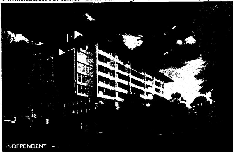
Figure 4 Jamieson Apartments Constitution Avenue Reid
