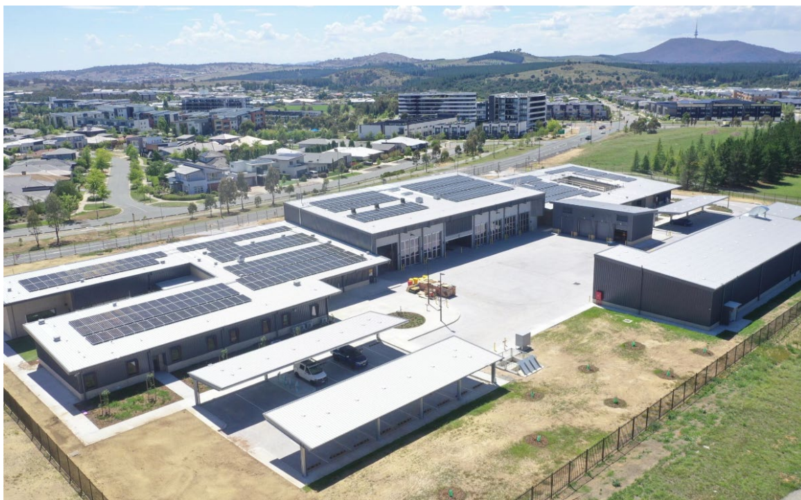
Recently Completed Molonglo Emergency Services Station
