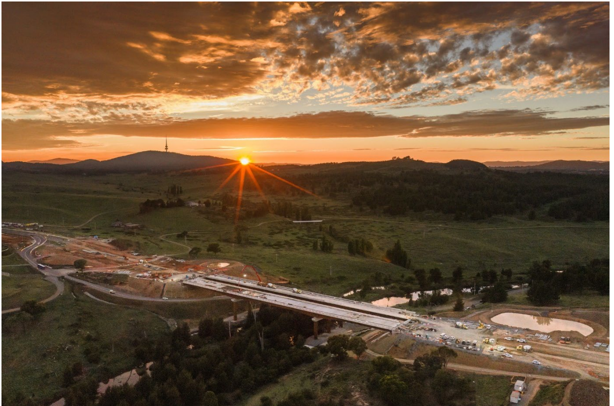
Molonglo River Bridge
