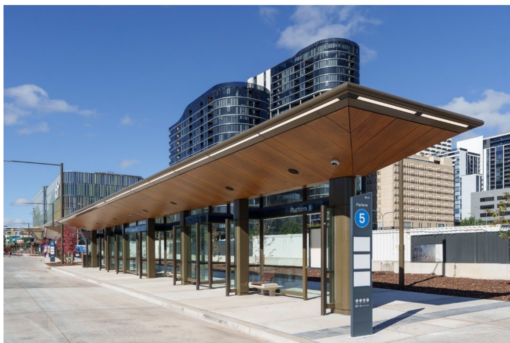
CIT Woden Transport Interchange
