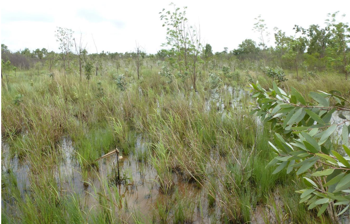
Figure 5. Wetland (Bellamack NT) establishing offline (with a lowered water level while plants establish)
