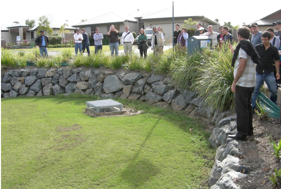
Figure 7. This bioretention system (Coomera Waters Qld) has been installed with a temporary cover of geotextile and turf to protect the filter from construction stage sediment (but still provide an attractive landscape outcome during the house-building phase)
