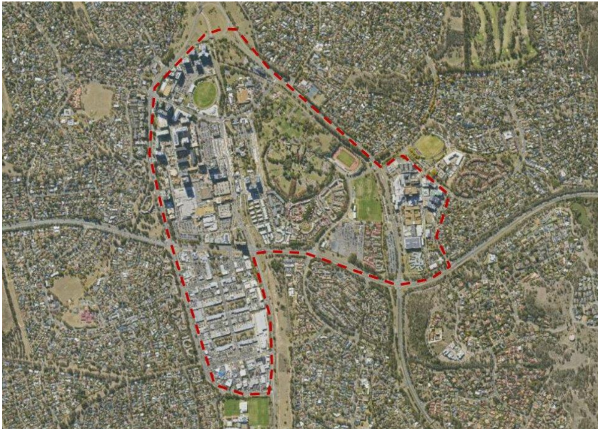
Figure 1 Woden Town Centre and surrounds
