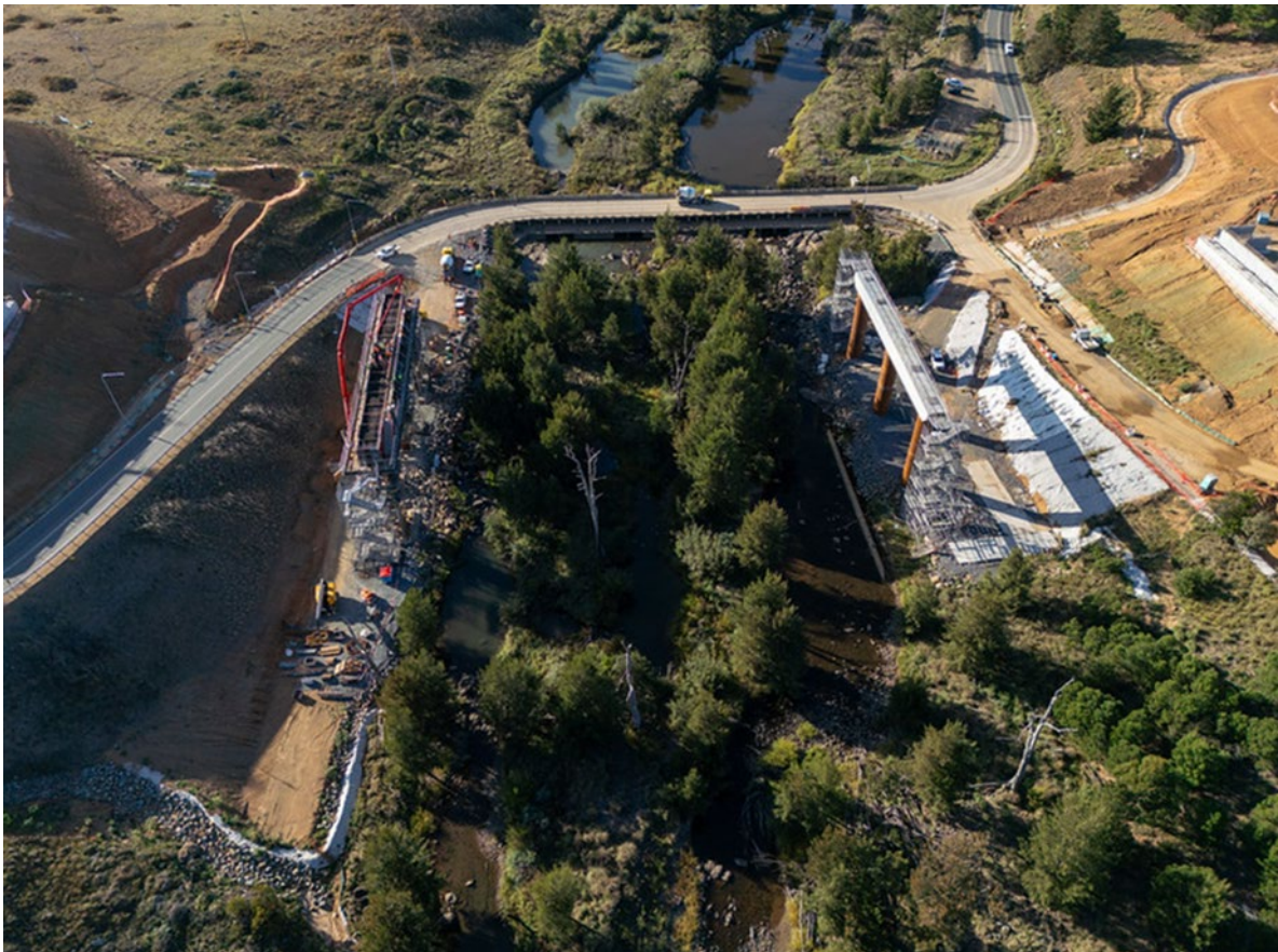
Molonglo River Bridge
