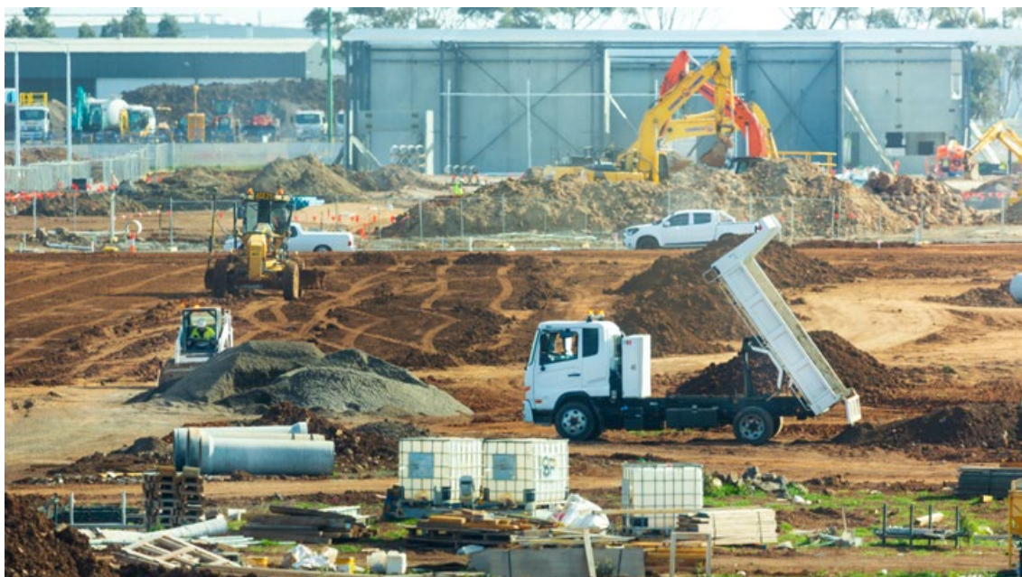
Construction in Victoria. Source: Troy Mortier
