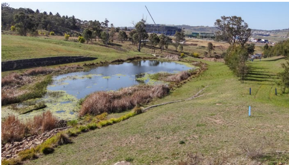
Urban stormwater in Denman Prospect. Source: OCSE
