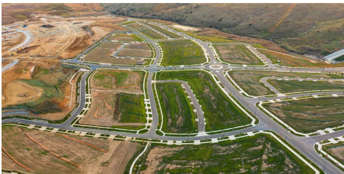
Whitlam under construction. Source: EPSDD
