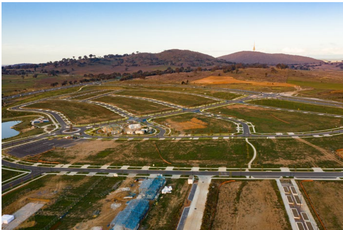
Whitlam under construction. Source: EPSDD
