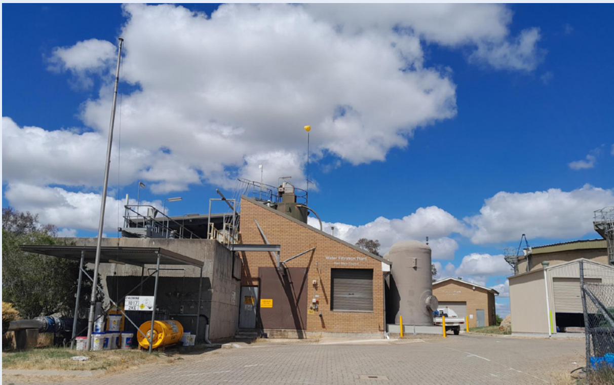
Yass Water Treatment Plant Photo credit: Yass Valley Council
