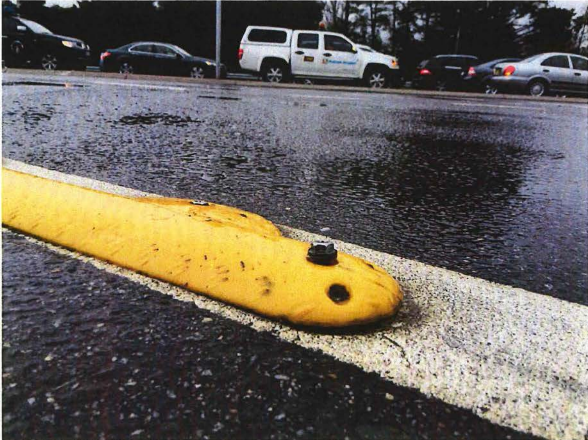
Figure 5. 12 months after installation
