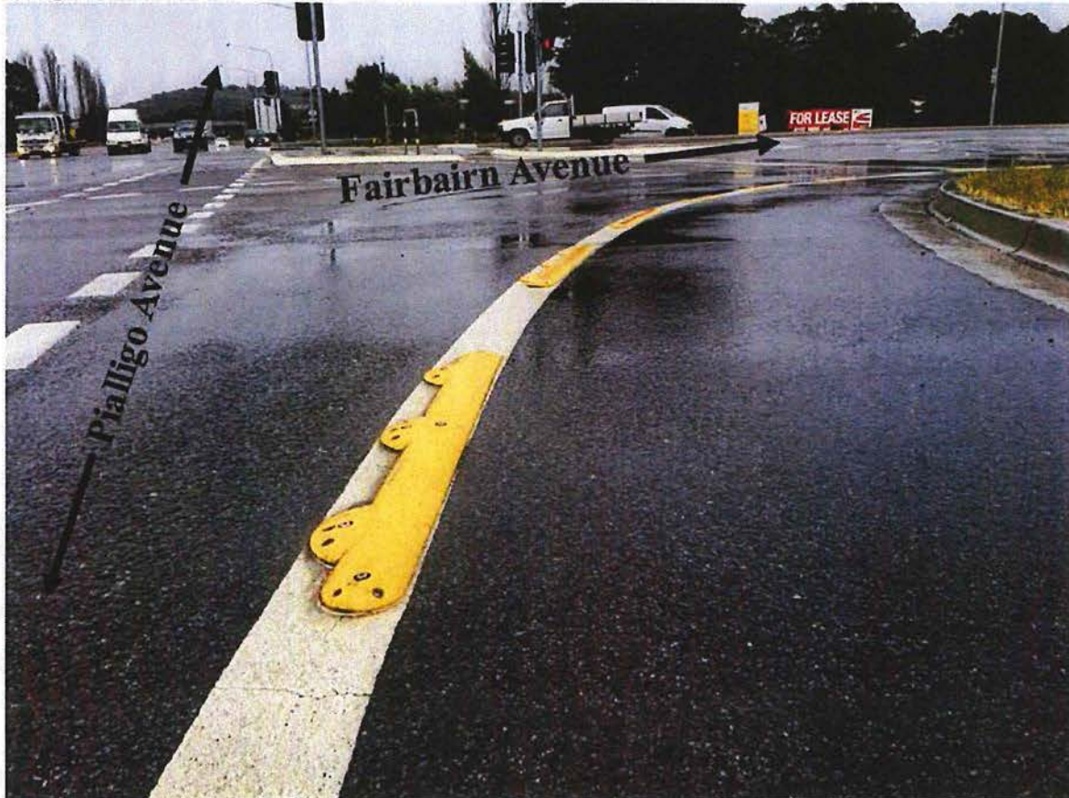
Figure 4. 12 months after installation
