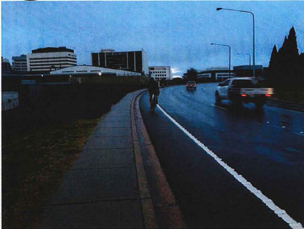
Figure 14. Scribed applied ATLM – 12 months after installation
