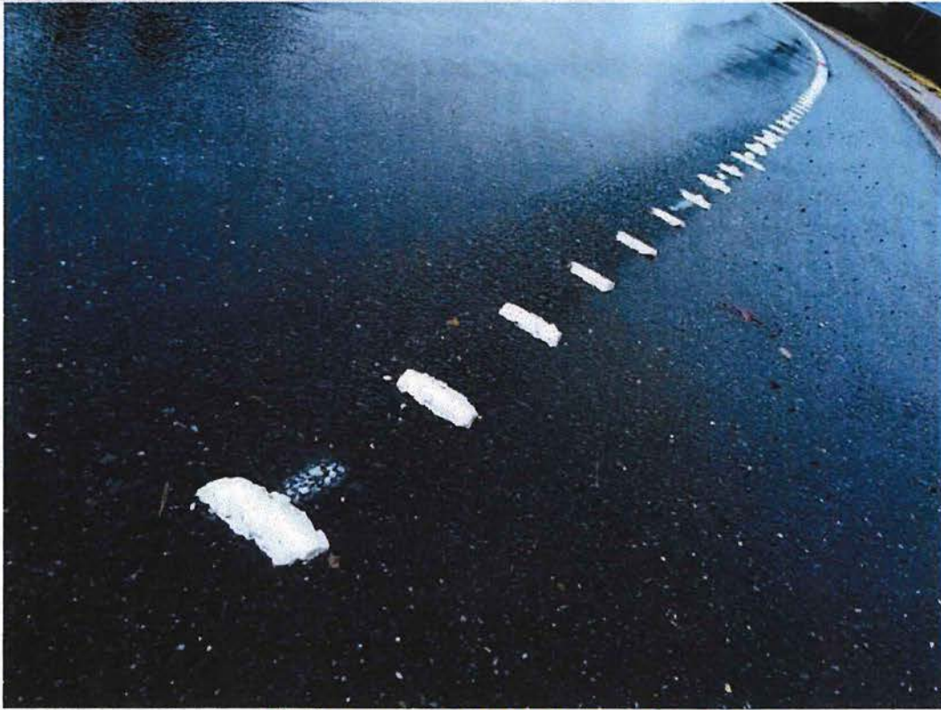
Figure 8. Screed applied ATLM – 12 months after installation
