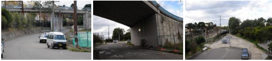
Figure 6. Sandwiched between the railway and highway, Katoomba skatepark suffers its location.
