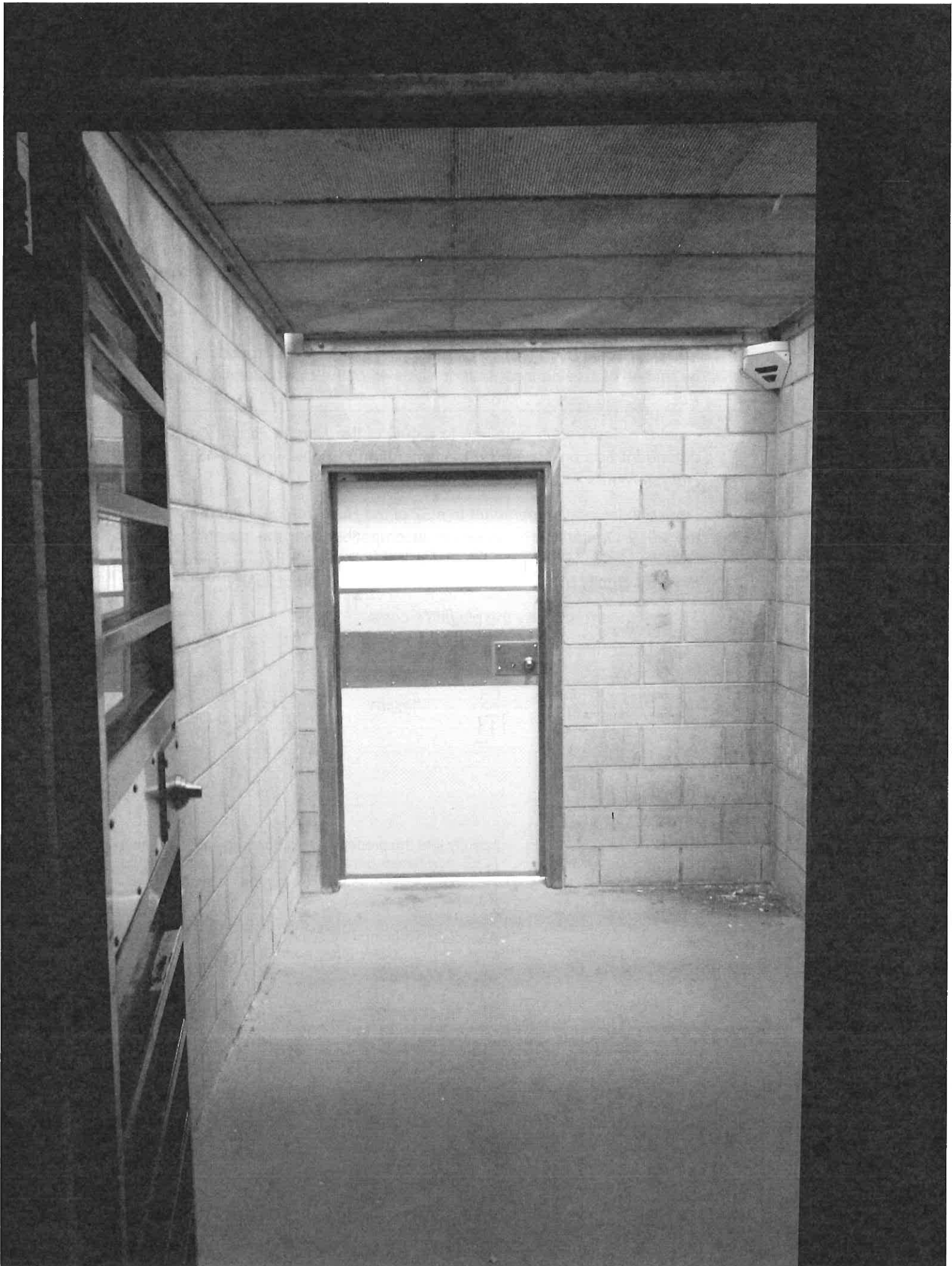
Annexure A: photographs of a rear courtyard and "hard side" cell exhibited to the affidavit of Mr Rust
