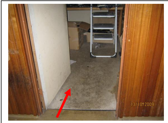
Photograph 1: Storeroom adjacent to bar – Vinyl floor tiles (refer sample 5038 – A3)
