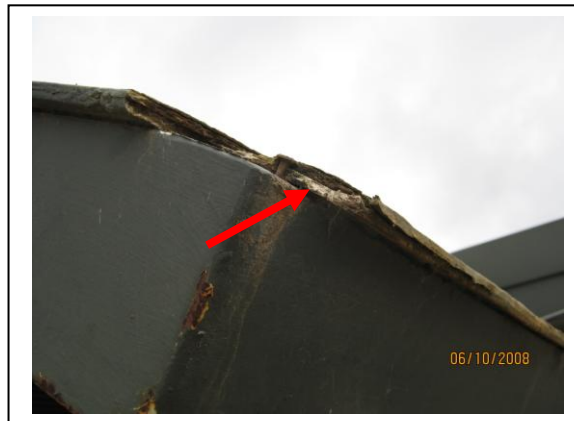
Photograph 9: Ground floor external – Sheet to awning above entry doors (refer sample 5038 – A14)
