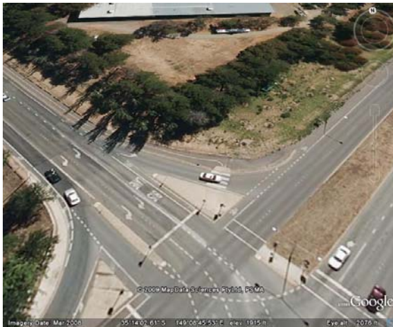
Flemington Road Mitchell showing Bus lane and Priority right hand turn
