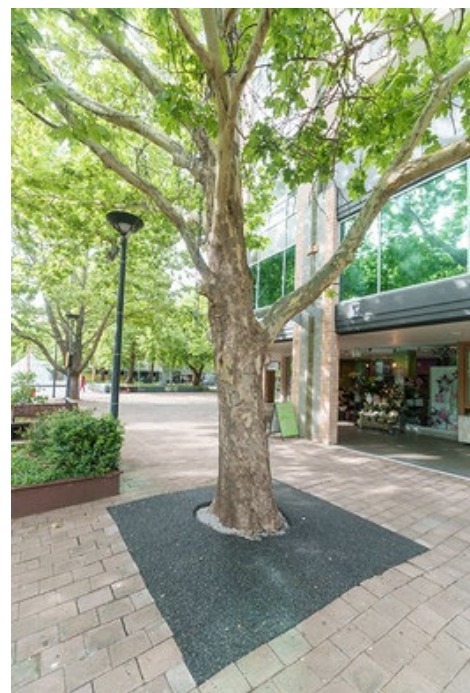
Image 11 City Walk permeable paving repair
