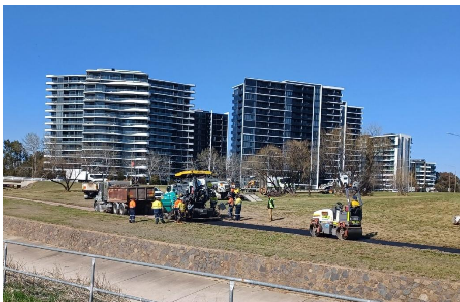
Re-surfacing the C4 at Yamba Roundabout
