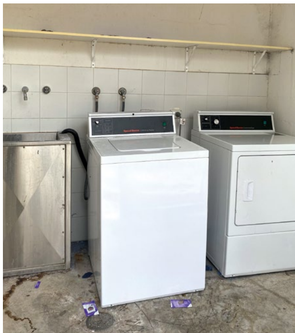
Photo 12: Accommodation unit laundry facilities
