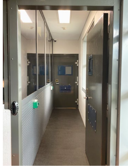
Photo 6: Corridor connecting the admissions side of Coree unit with the residential side
