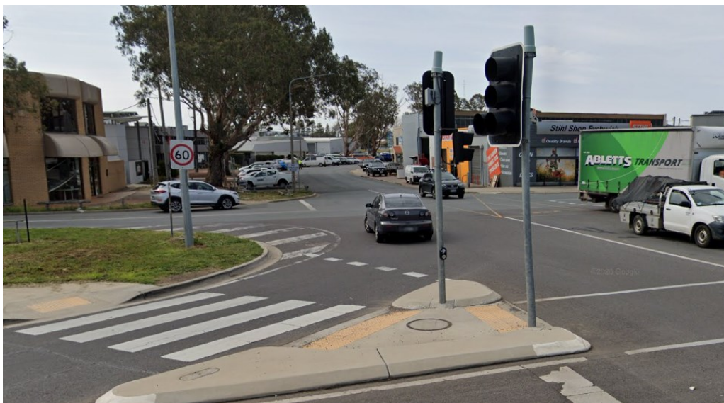
Figure 24: Incorrect speed limit signage on Geelong Street, captured by Google Street view in 2020. The signs were taken down, then reinstalled during intersection upgrades.
