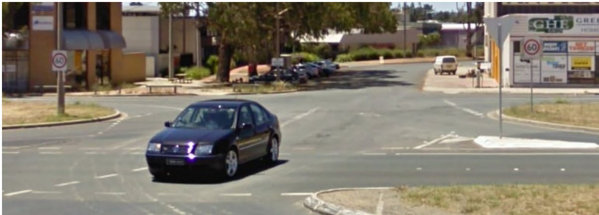
Figure 23: Incorrect speed limit signage on Geelong Street. Captured by Google Street view in 2009.
