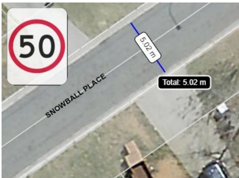
Figure 17: The road width of Snowball Place is only 5 metres wide but has an identical speed limit to several of Wanniasa's 17-metre-wide roads. If this had been the case due to the ACT trying to simplify urban area speed limits by setting a 50 km/h on every road and street in every residential area, then coming across two vastly different residential roads with an identical speed limit could have made sense. However as this was not the case. Therefore this situation does not make sense.
