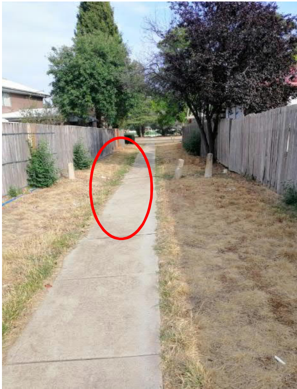
Figure 10 Missing bollard
