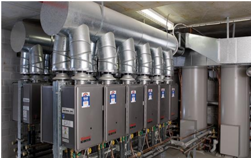
Figure 5: Typical multi-storey apartment block hot water system
