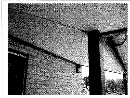
Photograph 2: Green Dormitory perimeter eave sheet Refer Sample: 5816 – A6
