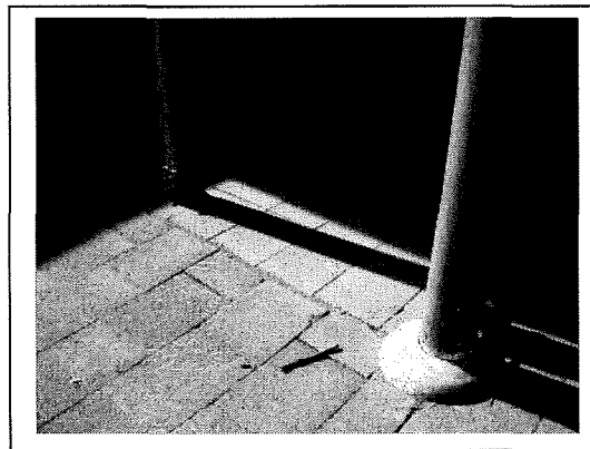
Photograph 8: Honyong courtyard verandah posts. 1 st Schedule Paint – 0.16 to 0.31% Lead Refer Sample: 5816 – P3(a,b,c)
